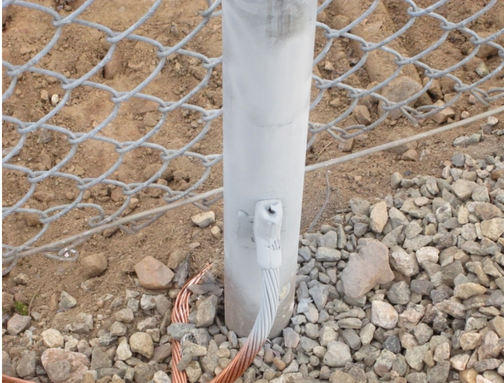
Figure 7: Typical grounding connection on terminal station fence
