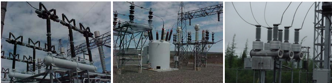
Figure 9: Circuit Breakers – ABCB (left), Oil (middle), and SF 6 (right)
