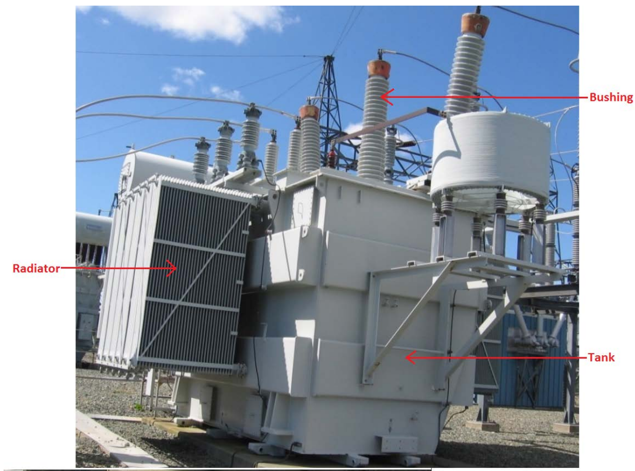
Figure 8: Power Transformer
