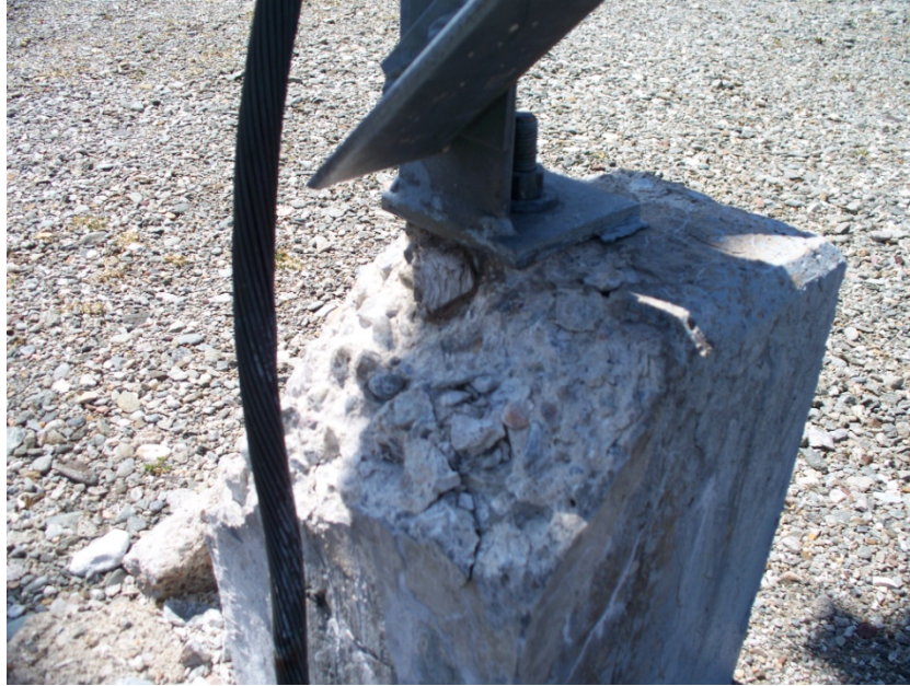
Figure 11: Structure B1T1 Bottom Brook Terminal Station
