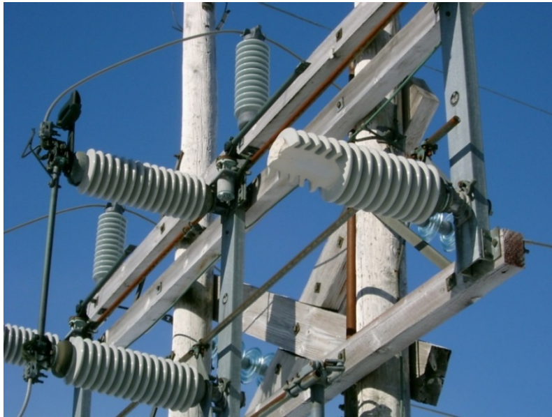
Figure 4: Broken insulator on 69 kV disconnect switch
