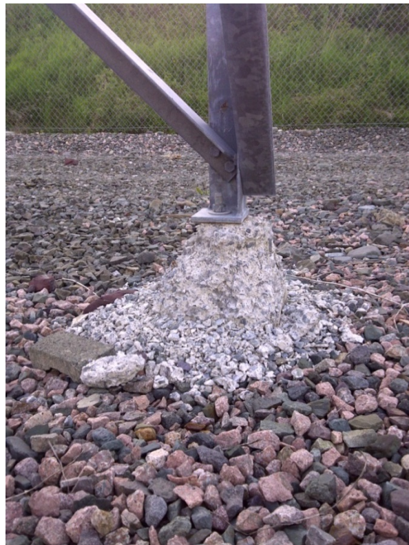
Figure 12: Structure L01L37-1 Western Avalon Terminal Station
