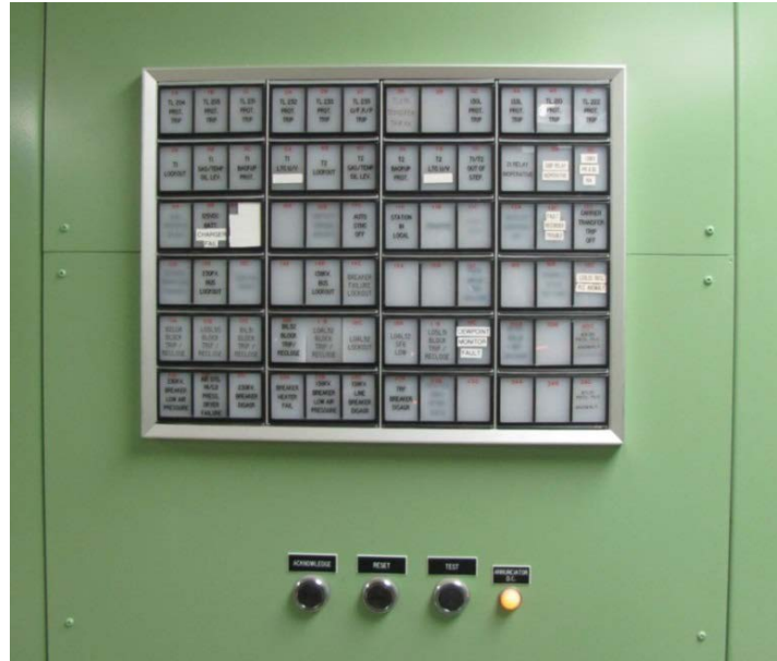
Figure 14: An annunciator commonly found in Hydro terminal stations
